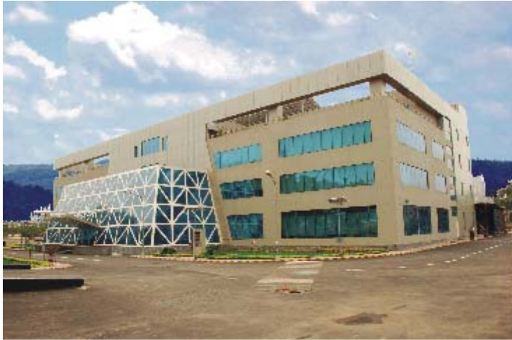
Switchgear Factory, Navi Mumbai
