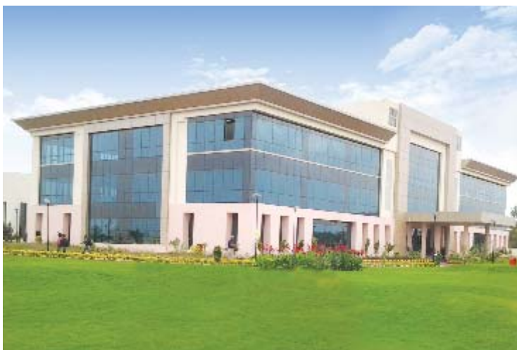
Switchgear Factory, Vadodara
