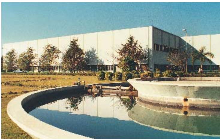
Switchgear Factory, Ahmednagar
